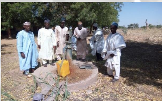
VHC members launching a repaired borehole water well in Banga PHC, Kaura Namoda LGA
